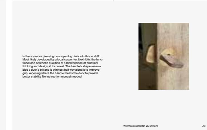
Is there a more pleasing door opening device in this world? Most likely developed by a local carpenter, it exhibits the functional and aesthetic qualities of a masterpiece of practical thinking and design at its purest. The handle's shape resembles a duck's bill and is thinnest half way along it to improve grip, widening where the handle meets the door to provide better stability. No instruction manual needed!
